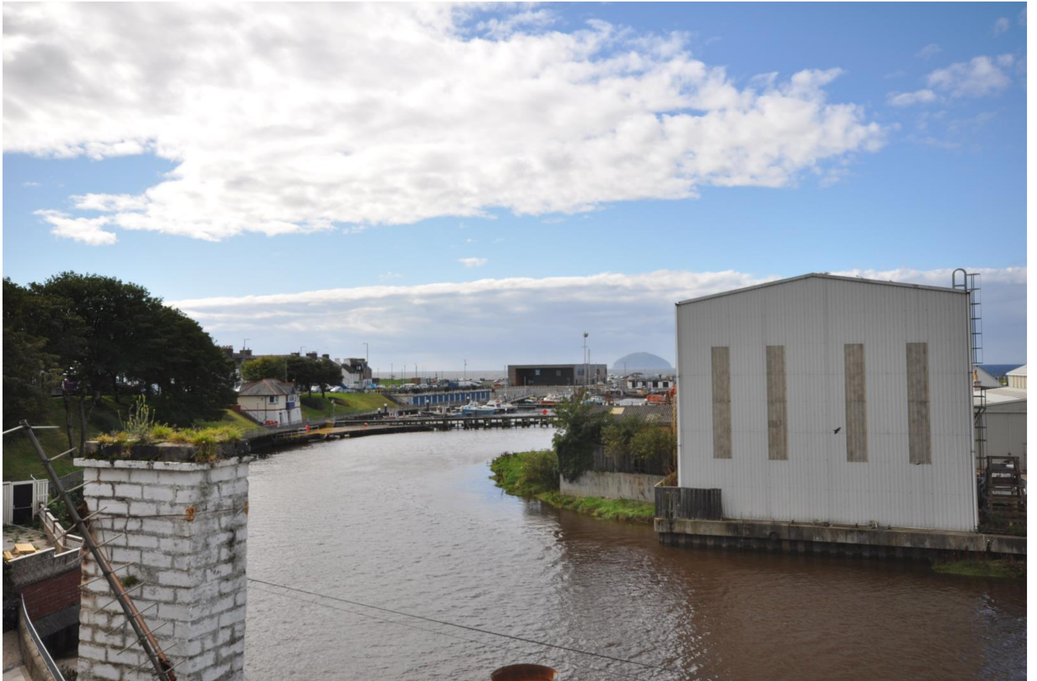
View from rear of property
