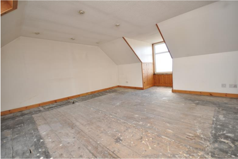
Room in the Roof 1
