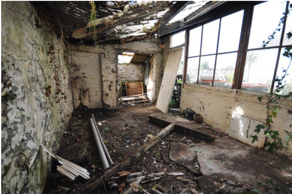
Space at rear of property
