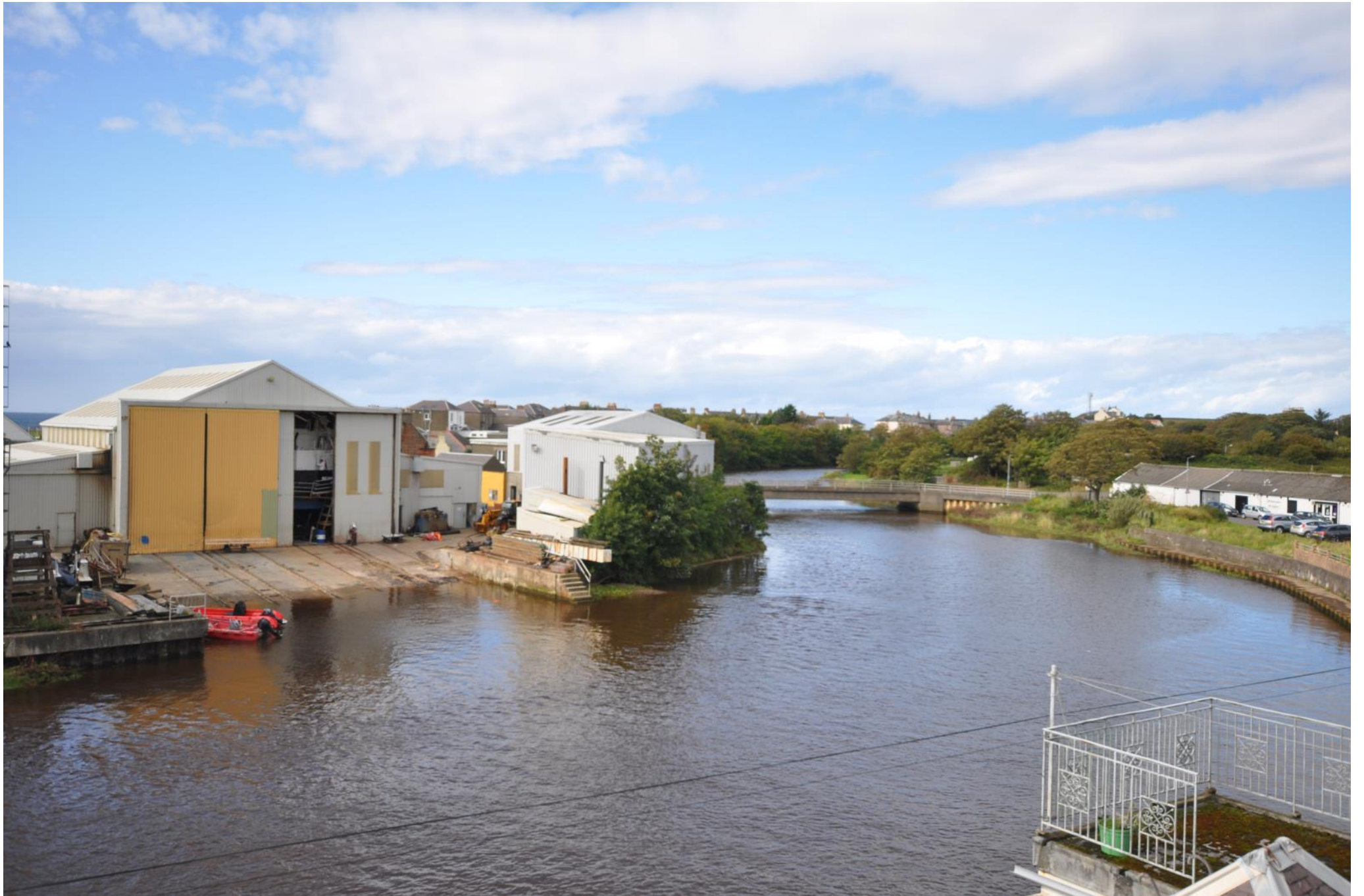
View from rear of property
