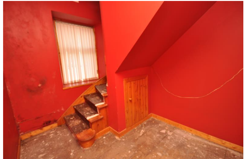
Stair to Rooms in the Roof
