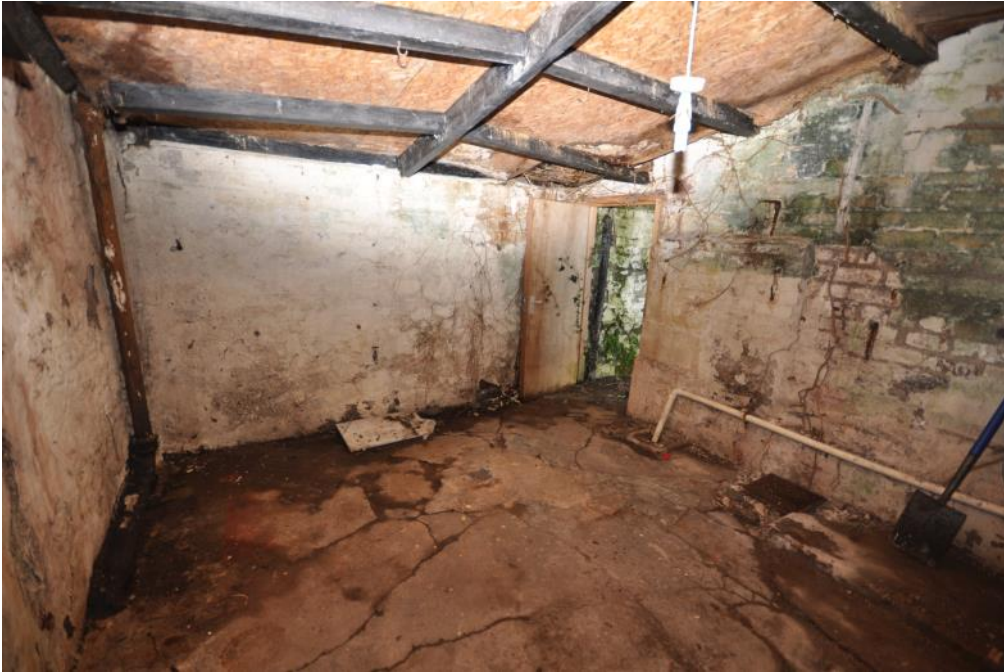
Space at rear of property
