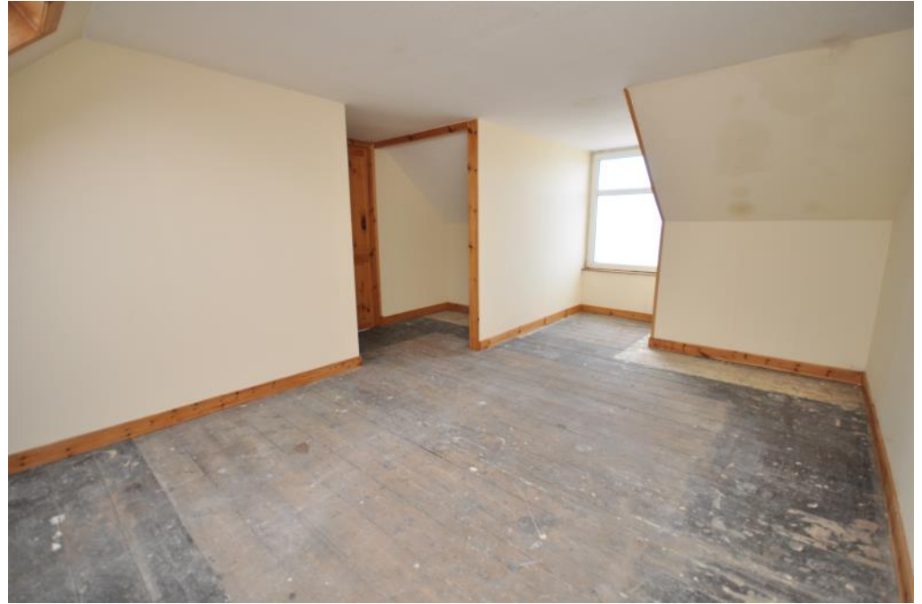
Room in the Roof 2
