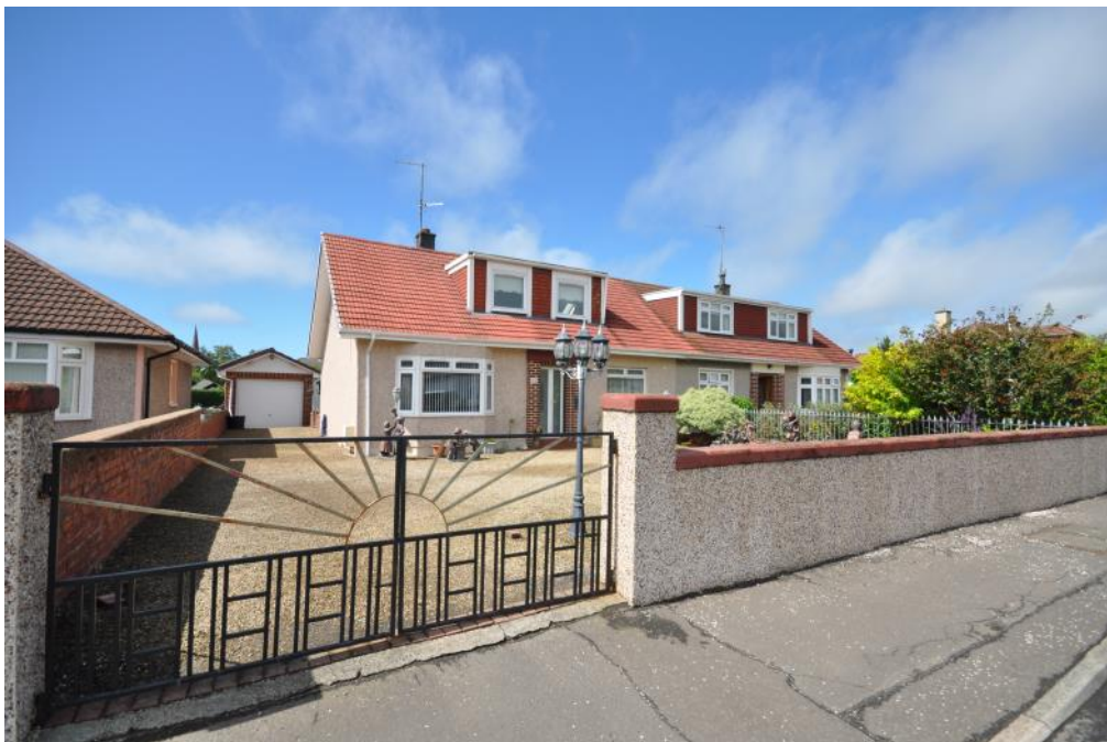
Front from street
