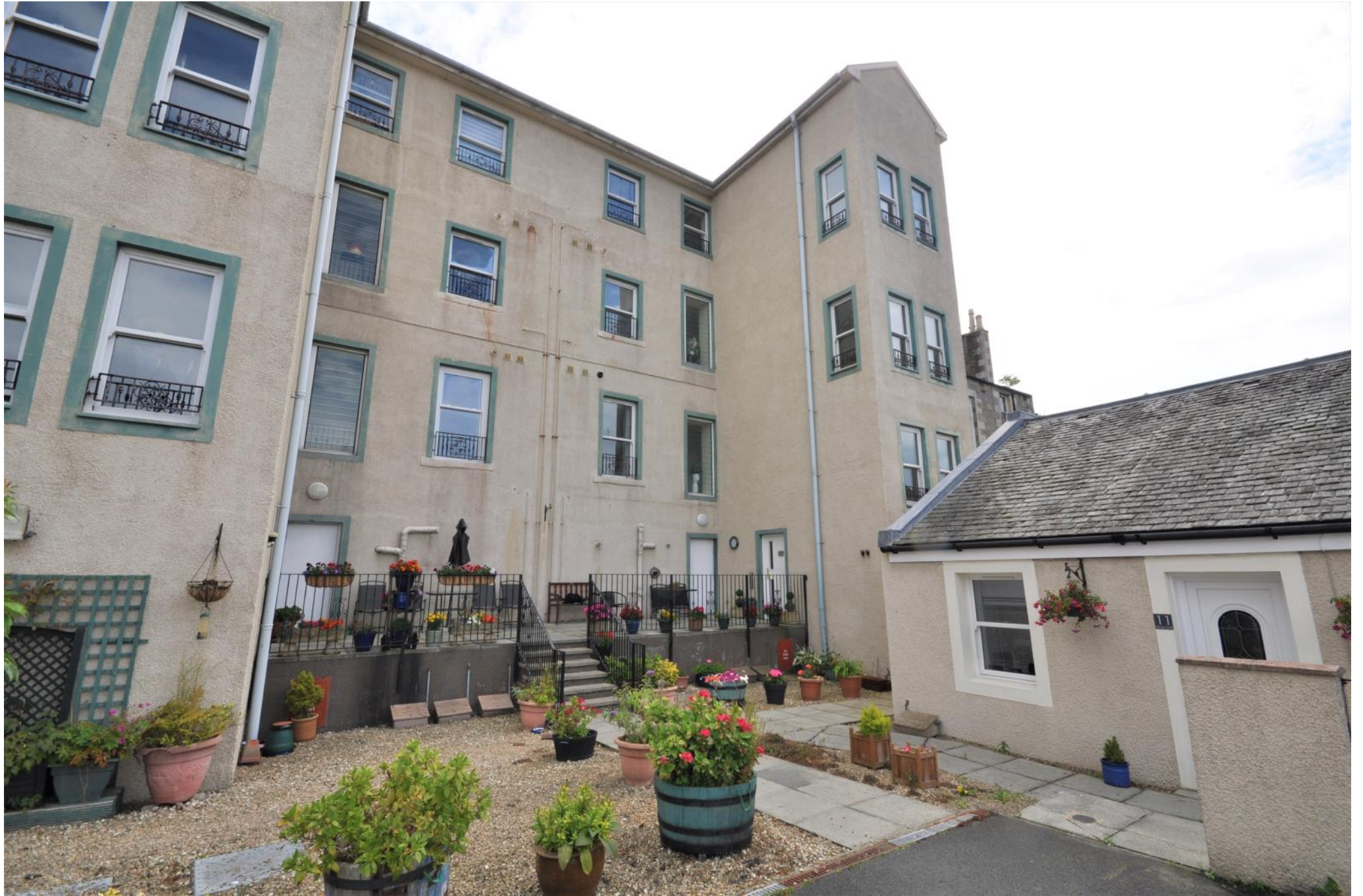
Back of Building
