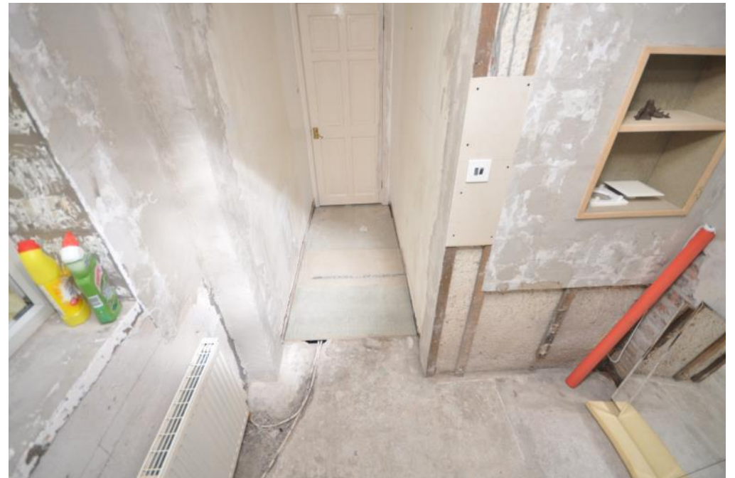
Space for Bathroom
