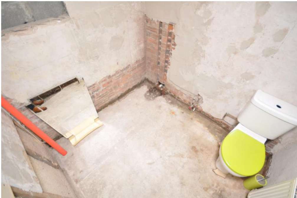
Space for Bathroom
