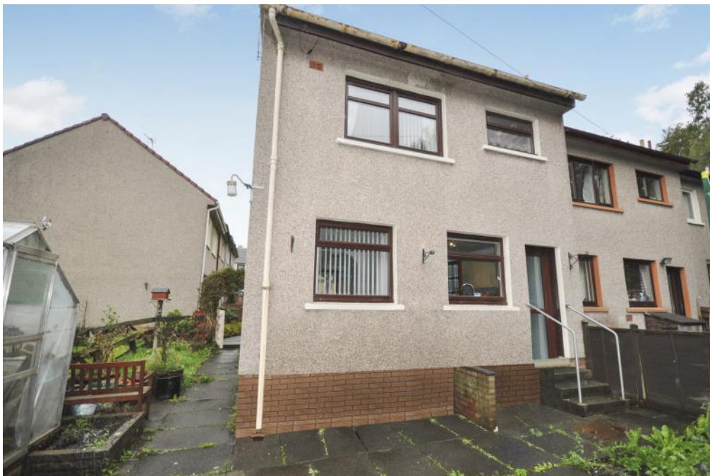
Rear of House
