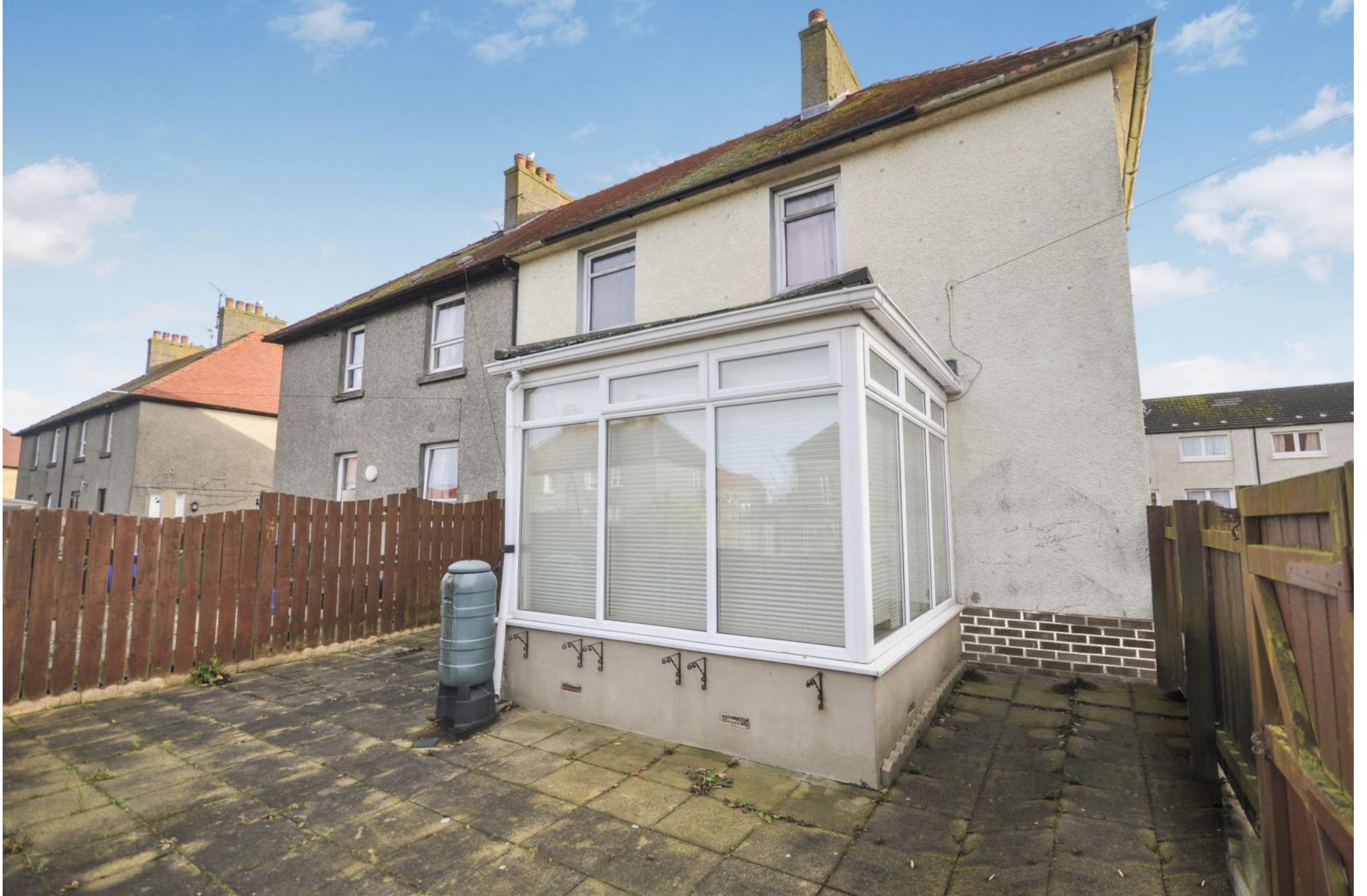
Rear Elevation and Back Garden
