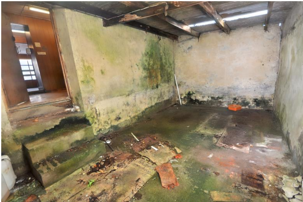
Covered Outside Area
