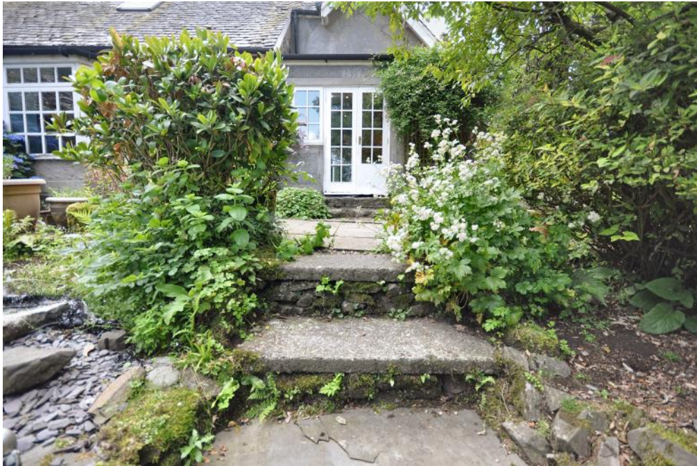
Steps down from terrace
