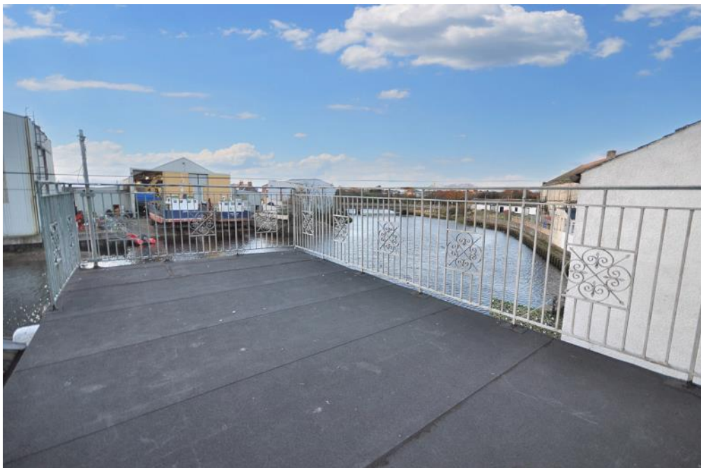
Flat Roof Space
